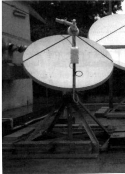
**Figure 9.30** Photograph of a C-band VSAT installation with a 2.4m antenna.
