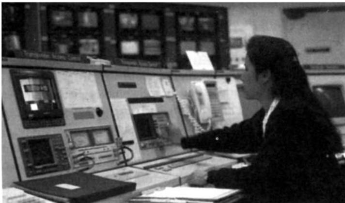
**Figure 9.22** The downlinks of the JC Sat satellites are monitored on a 24-hour basis by communications controllers at the JC Sat network operations center. (Source: Photograph courtesy of Sky Perfect JSAT, Ltd.)
