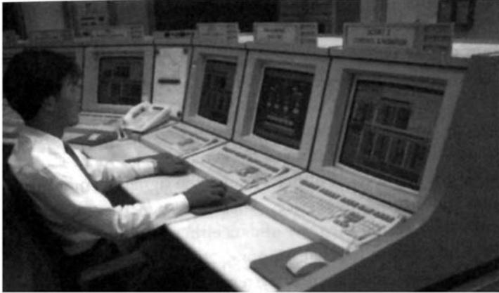
**Figure 9.21** The satellite control console where the JC Sat satellites are controlled and monitored through the video display terminals. The Yokohoma TT&C station is used as the primary operation center for the JC Sat systems. (Source: Photograph courtesy of Sky Perfect JSAT, Ltd.)
