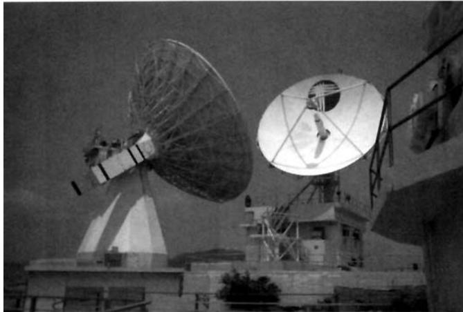
**Figure 1.15** This INTELSAT Earth station antenna in Hong Kong was built at 30m to be able to operate with low-power C-band satellites such as INTELSAT III.
